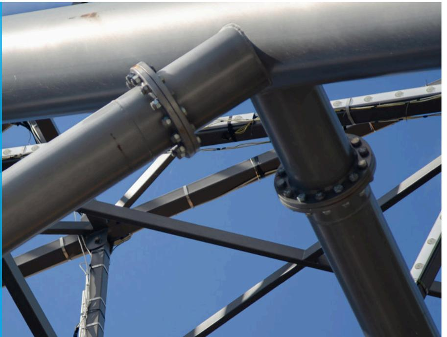
Expect simpler assembly, fewer errors, and optimized efficiency with our combi nuts, combining a nut with a pair of captivated Nord-LOCK original washers.
