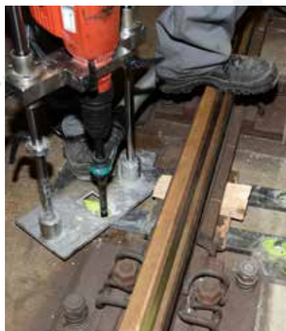
The rails of the Nuremberg underground are fitted onto longitudinal beams made of reinforced concrete using a rail mounting system, which is, in turn, connected to the tunnel floor. In recent years, the concrete stringers have been repeatedly damaged. The new concrete bolts are fitted with a patented special thread that cuts into the borehole wall upon application.
