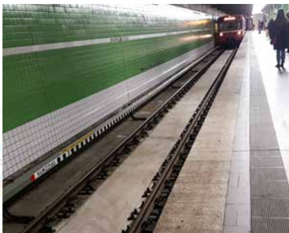
The rails of the Nuremberg underground are fitted onto longitudinal beams made of reinforced concrete using a rail mounting system, which is, in turn, connected to the tunnel floor. In recent years, the concrete stringers have been repeatedly damaged. The new concrete bolts are fitted with a patented special thread that cuts into the borehole wall upon application.
