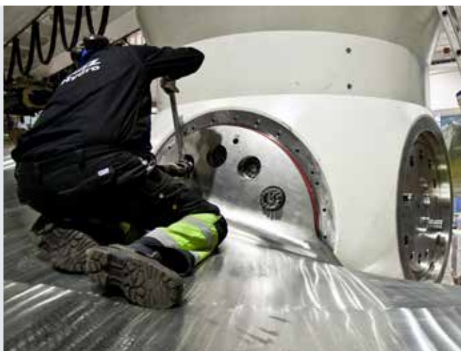
Åsa Eklund, System Engineer for the refurbishment of Laxede power station, believes that the SB12 bolt-style Superbolt tensioners from Nord-Lock, which they are using for the first time, have worked well. The bolts are attached to the blades and the runner – see picture to the left.
